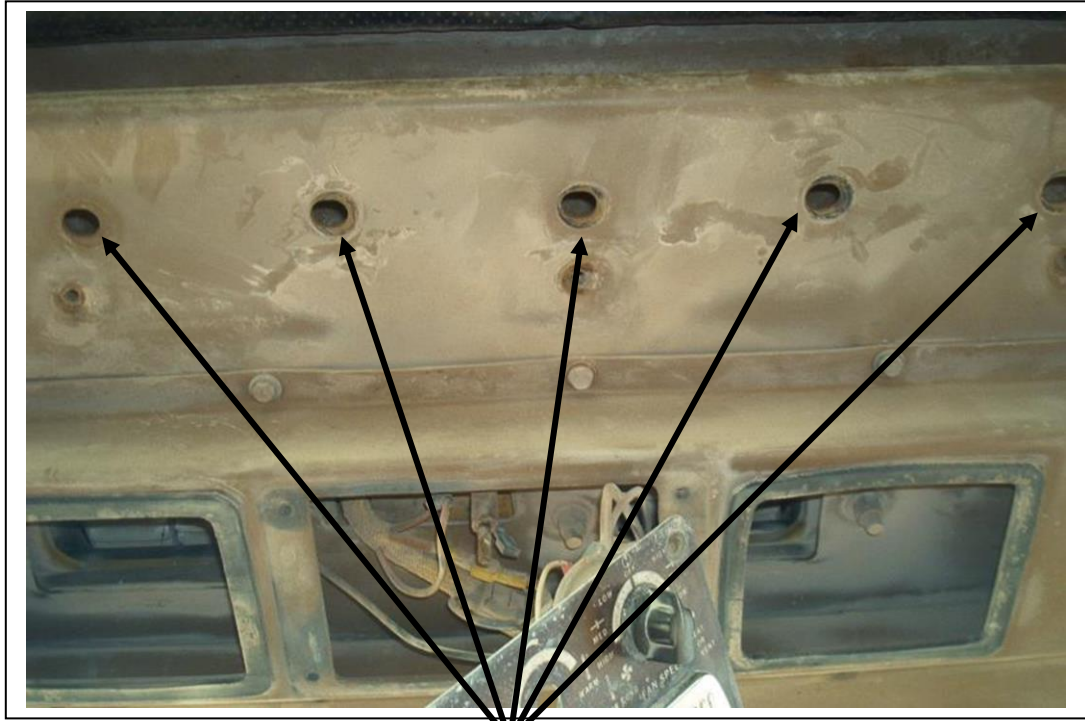
Bolts removed to lower heater box.
