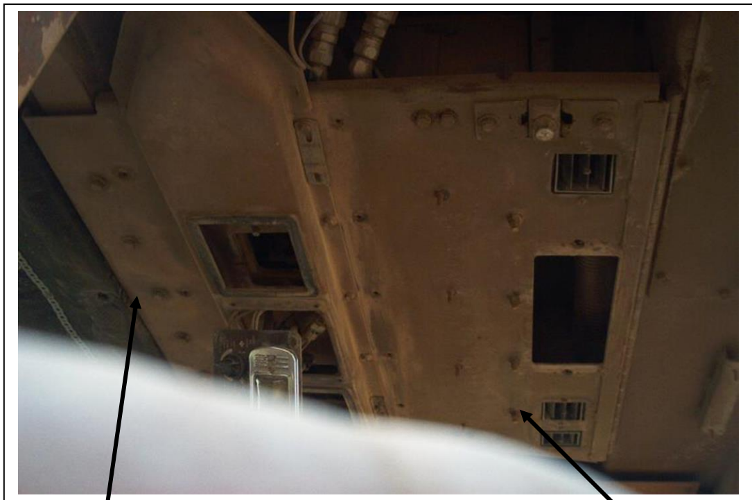
Removed these 5 bolts
